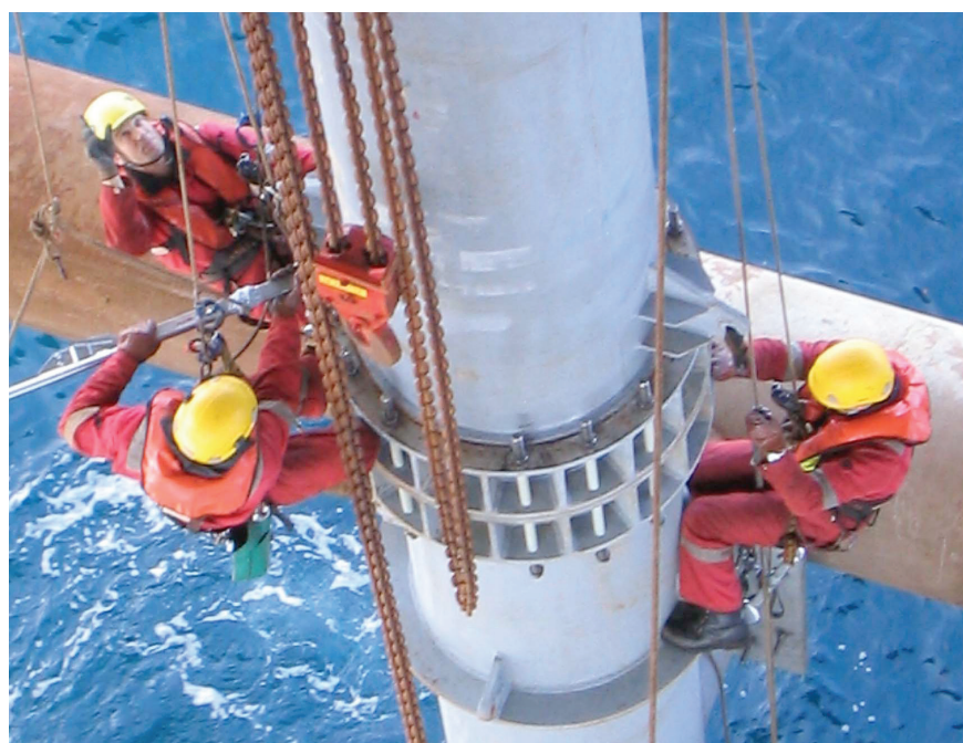
Operations such as rope access are categorised as high risk. Photograph: CAN Group.
